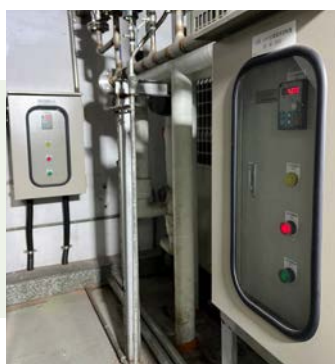
Windmill plug-in inverter in Zone 06
