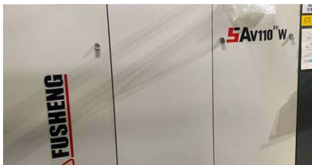
▲ 07 Area – Replacement of air compressors
