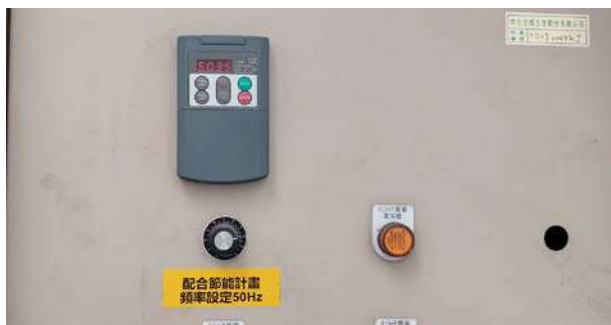
▲ 60HZ frequency of 60HZ ventilator of the Occupational Safety and Health Department was adjusted to 50HZ
